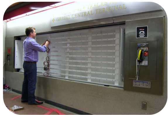
Matrix in place
