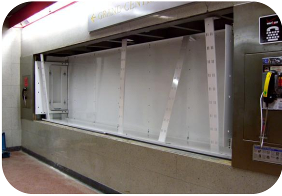
Ready for installation
